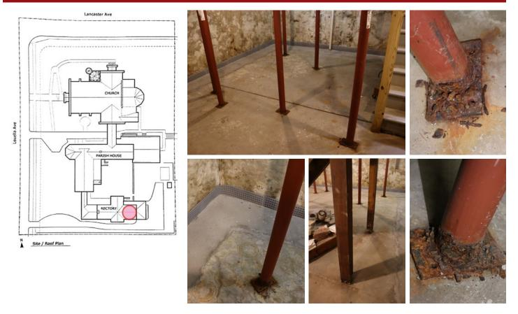
Issue: Persistent flooding has caused deterioration of lally columns and wood posts
