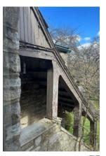
Issue: Joint in copper gutter has been leaking for years, extensive water/rot/insect damage to crown molding, eave, T&G siding, and timber frame of fire exit stair roof canopy.
