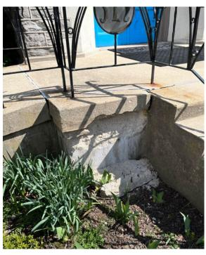
**Issue**: Moisture has penetrated the upper landing slab at the railing post penetrations, spalling has broken off a large chunk below the slab, cracks and rust staining visible in slab.
