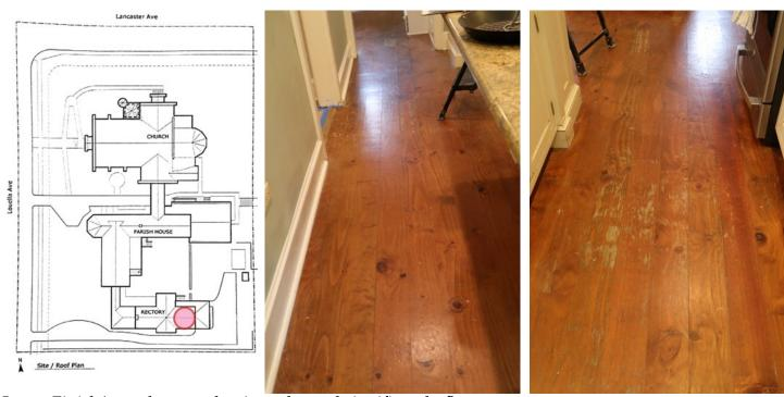
**Issue**: Finish/wear layer on laminated wood significantly floor worn. **Solution**: Remove and replace in kitchen and laundry, selection TBD.
